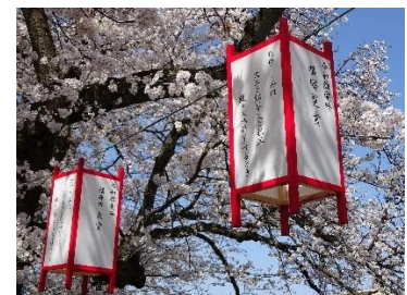
足羽川左岸堤防
